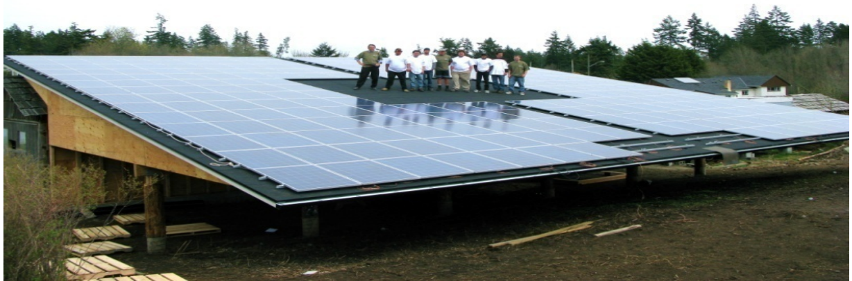
Figure B.1.b: 39.9 kW Canoe shed PV system. Image from Bekker (2009a, 24).
