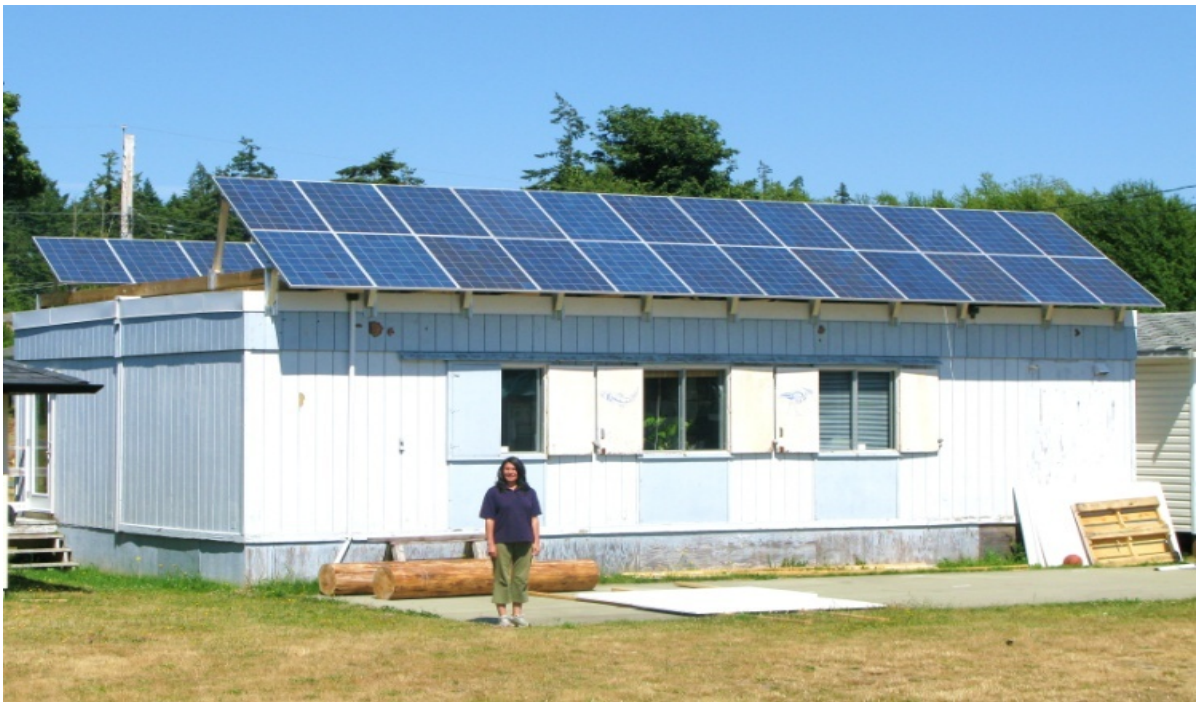
Figure B.1.e: 6.3 kW Fisheries PV system. Image from Bekker (2009a, 7).
