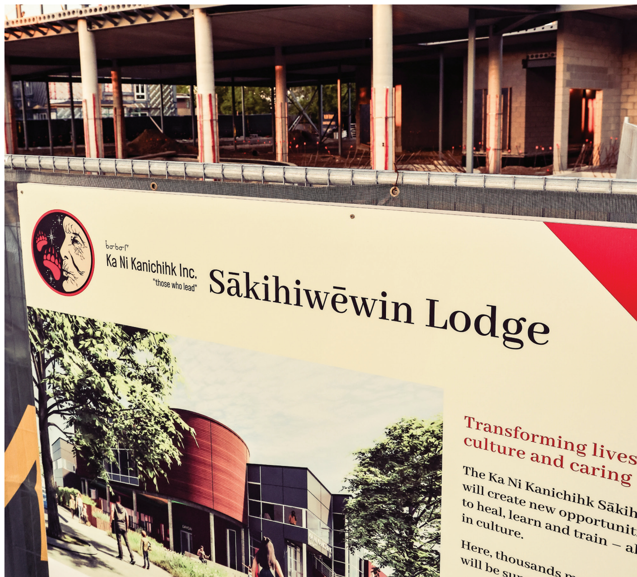
PHOTO 2 Sākihiwēwin Lodge under construction
