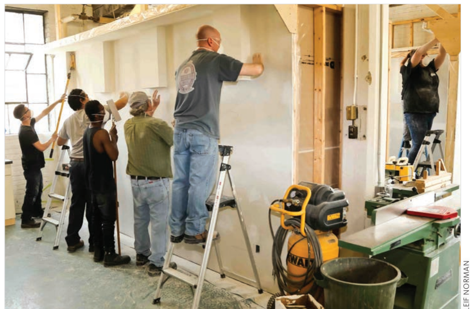
Trainees at BUILD learn patch and paint techniques.
