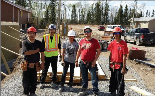
ATEC students on the worksite in Nisichawayasihk Cree Nation.
