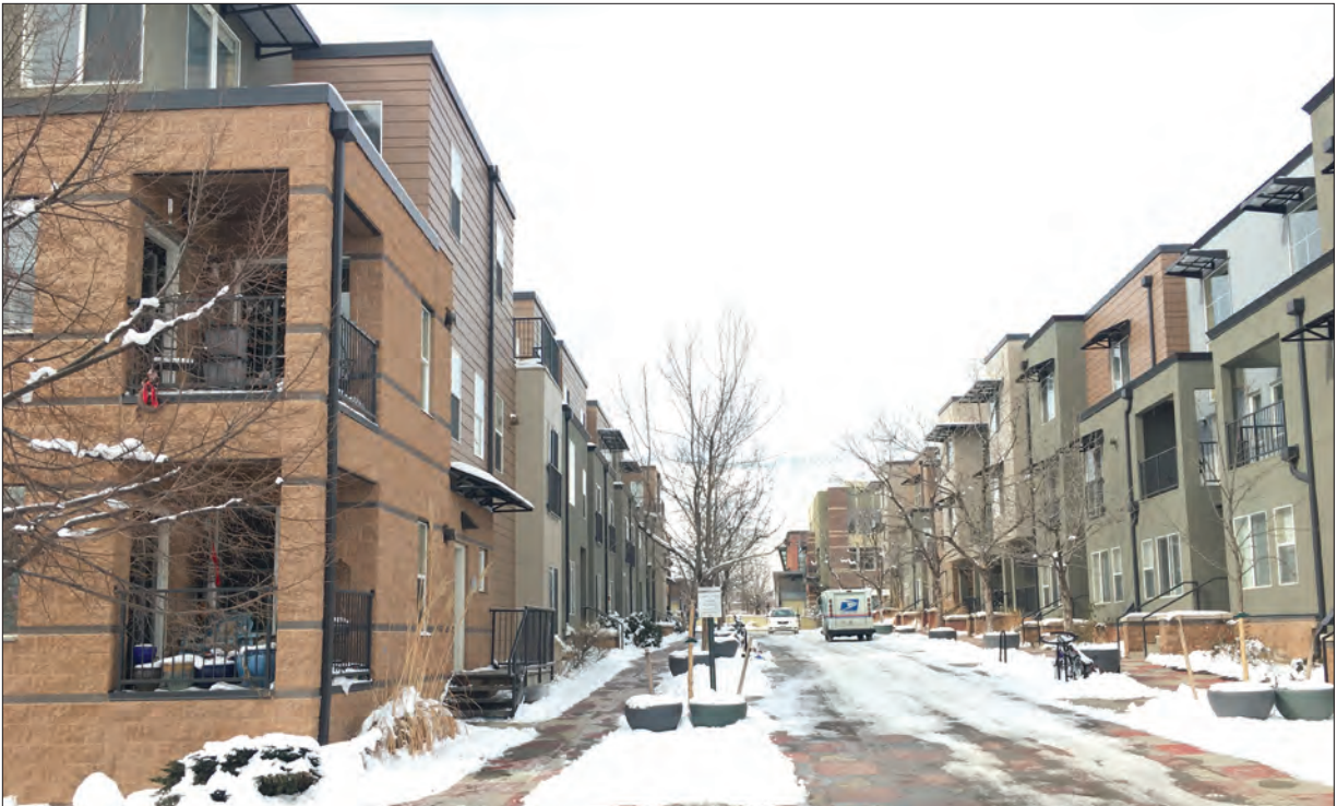
FIGURE 2 New Mixed-Income Housing Development
