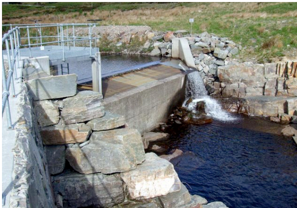
Cuileig run-of-river hydro plant in Scotland.
