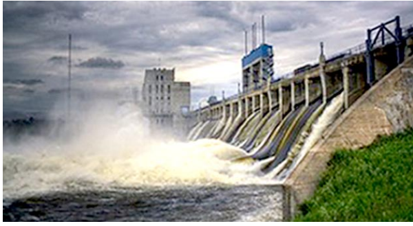
Seven Sisters Hydroelectricity Dam – Manitoba
