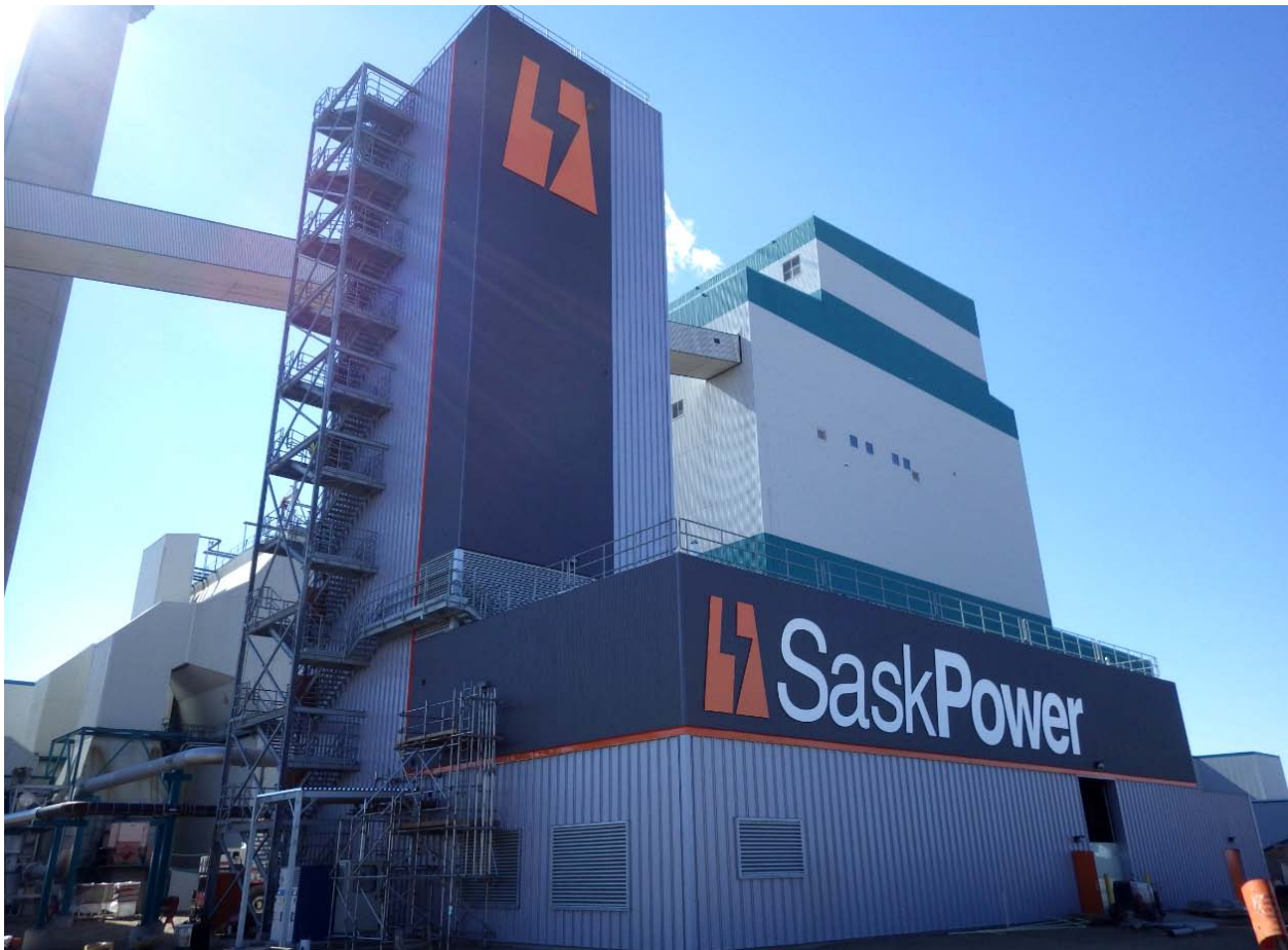
Shand Carbon Capture Test Facility
