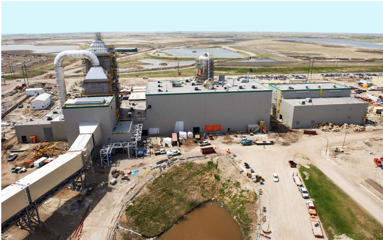
Boundary Dam CO 2 capture plant
