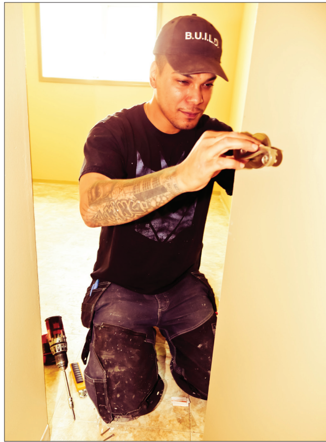
BUILD trainee at work
