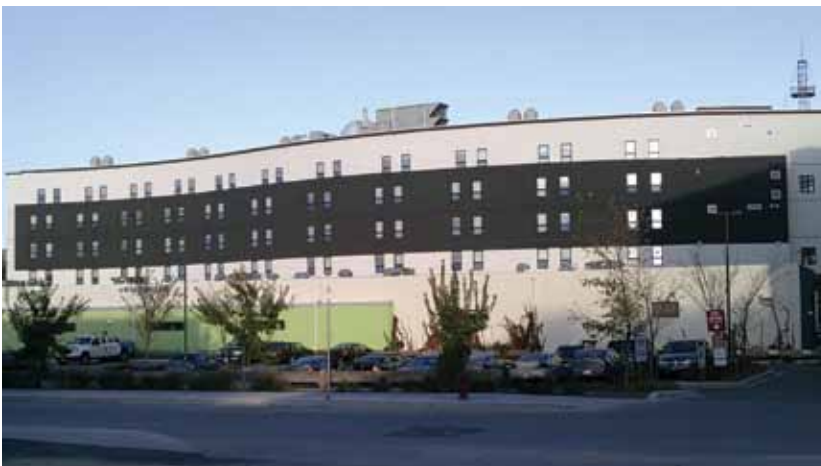
PHOTO 34 Picture of the Back of Building
