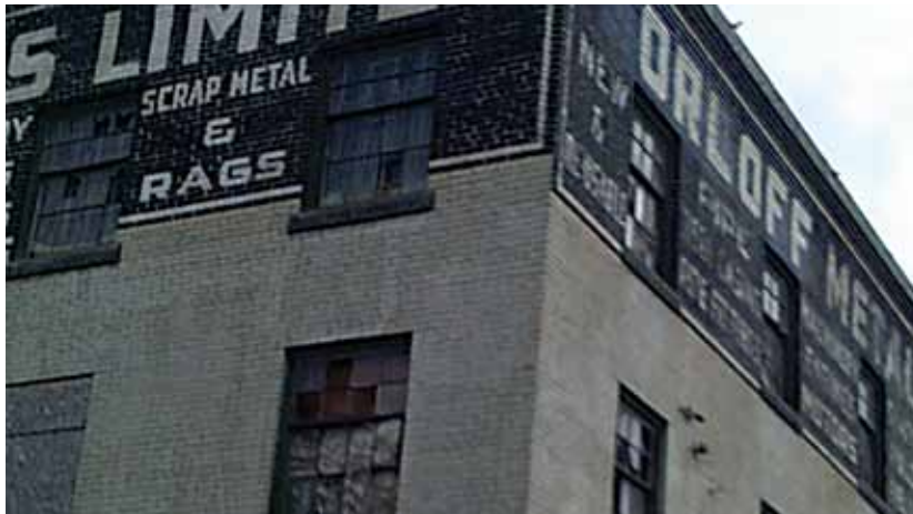
PHOTO 24 Old Warehouse Building on Stella Ave at Main
