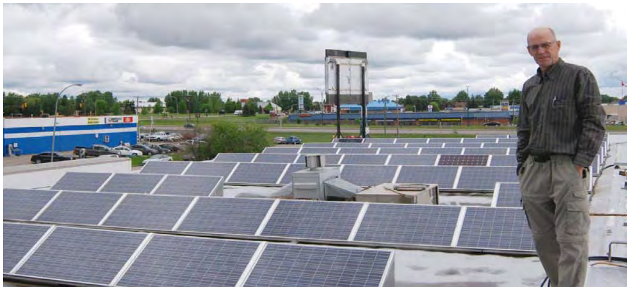
Since purchasing the Confederation Inn in Saskatoon in 2006 Brian Sawatzky has steadily reduced energy and water consumption in his business. He has installed a solar hot water system and a solar photovoltaic system, along with triple pane windows, improved insulation and LED lighting. He is saving over $130,000 per year on his utility bills, and has now achieved nearly a 70% reduction in energy use. His greenhouse gas reduction is approximately 460 tonnes CO 2 e (carbon dioxide equivalent) per year. Brian Sawatzky’s leadership example illustrates the potential direction that could be taken by thousands of other businesses across Saskatchewan. (Photo Credit: Lynette Suchar; Photo Location: Rooftop of the Confederation Inn; GHG reduction estimate: Special thanks to Angie Bugg.)
