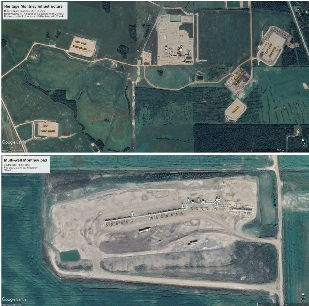
Figure 12: Multi-well pads in the Heritage Montney field.
